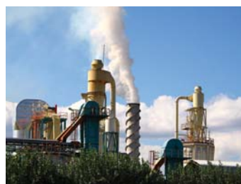
Steam exhaust from power plants
